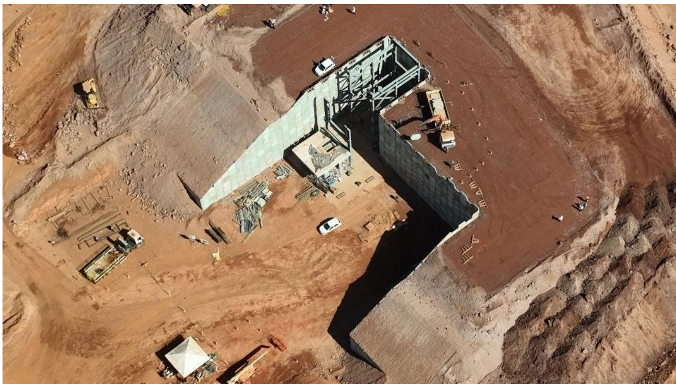
Figure 4: Construction of primary crusher retaining wall at the Tucumã Project (July 2023).
