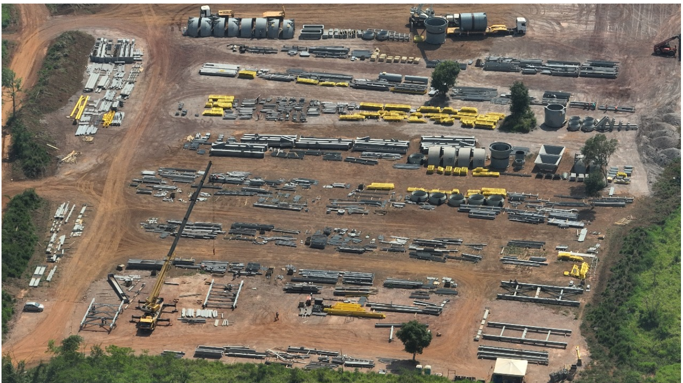
Figure 7: Project laydown area for pre-assembly and steel storage.
