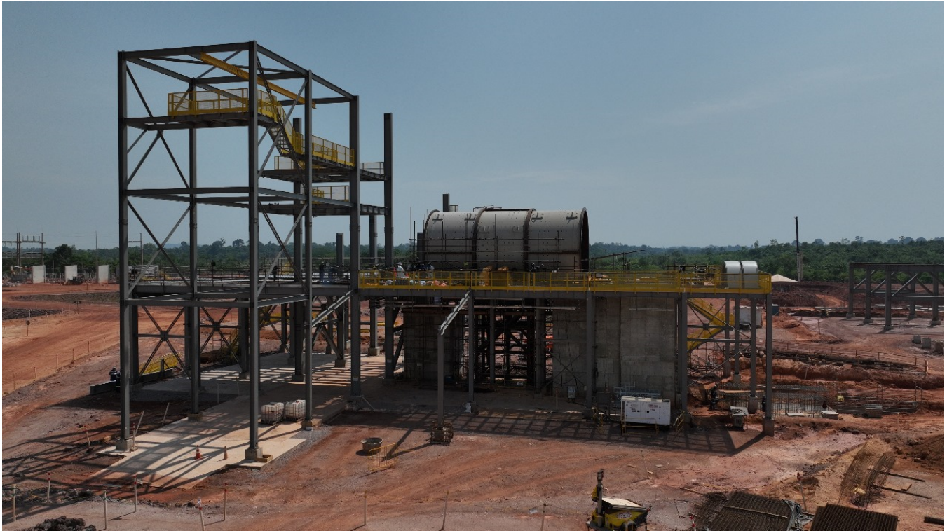
Figure 2: Installation of the Ball Mill for the Project.
