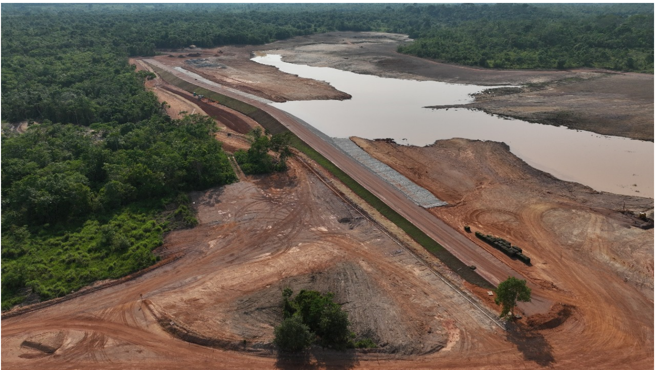
Figure 5: Completed water reservoir.
