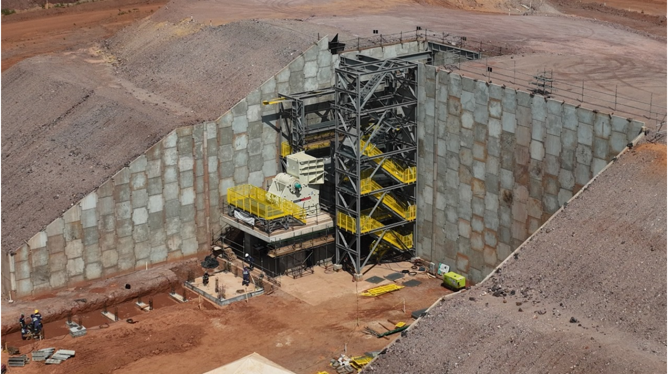
Figure 4: Installation of the primary crusher.
